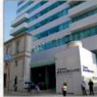
Nova Torre (Bloco A) Hospital Bandeirantes
